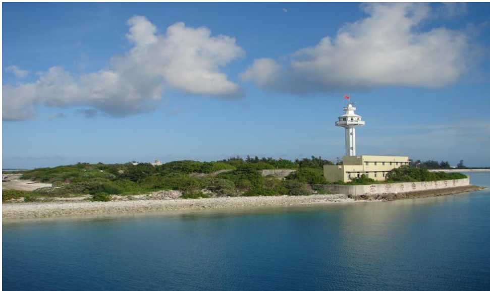
Duncan, Communication Tower
